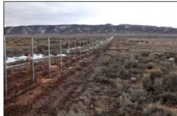
Border fence construction is complete
